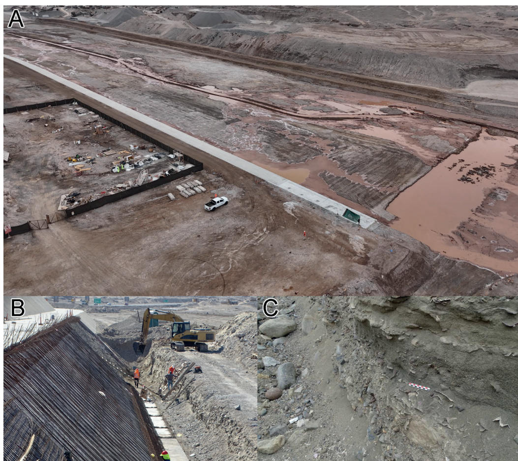
Figure 10 - Exposure of shelly beds found during public works excavations, Río Salado. A) Aerial view following rainfall 02/2026. B) River floodwall construction. C) Fossiliferous outcrop
